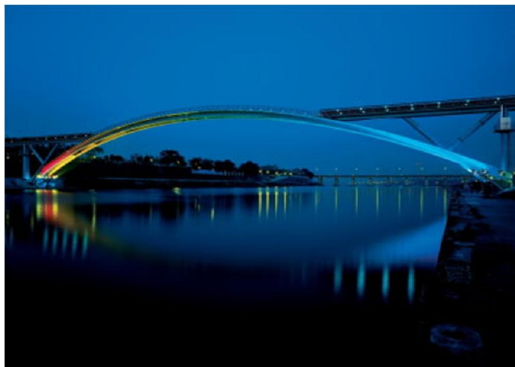
Seoul bridge, South Korea
